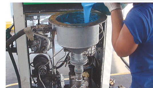
▲ Inner pipe coating
